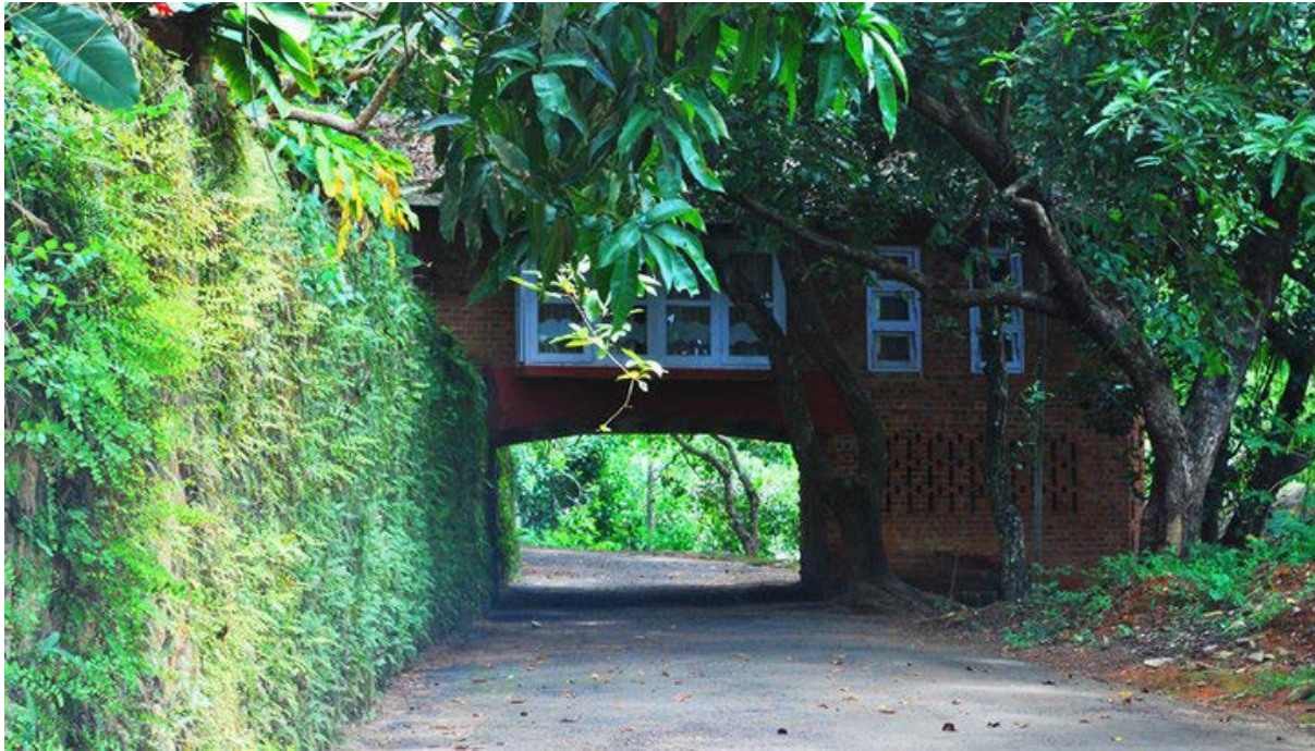
Figure 6: Entrance Building at Centre for Developing Studies, Trivandrum (Source: Author)
