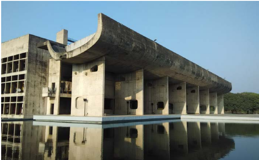
Figure 1 Le Courbusier's Architecture, Capitol Complex, Chandigarh (Source: Author)
